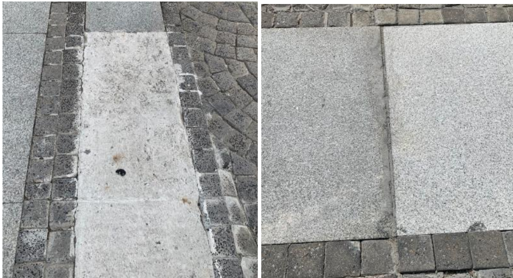
Figure 58: Granite Replacement: Quality issues
