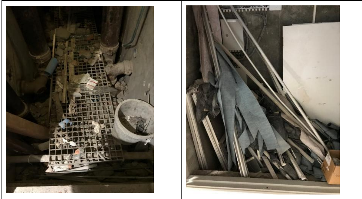
Figure 56: 90 Plein Street - 6th floor refurbishment: Quality issues
