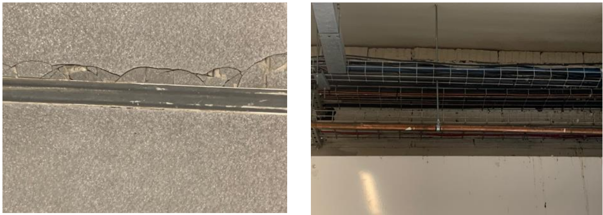
Figure 57: Swans Garage: Quality issues
