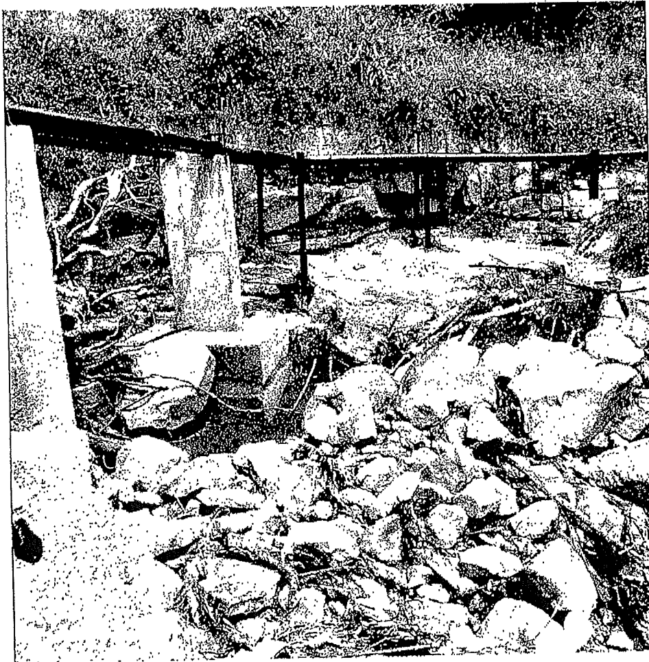
Figure 11: Bridge to sludge drying beds to be reconstructed
