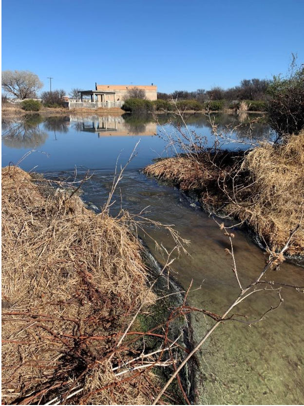
The Meloding sewage plant is in an advanced state of decay and all the sewage flows into local rivers and streams.
