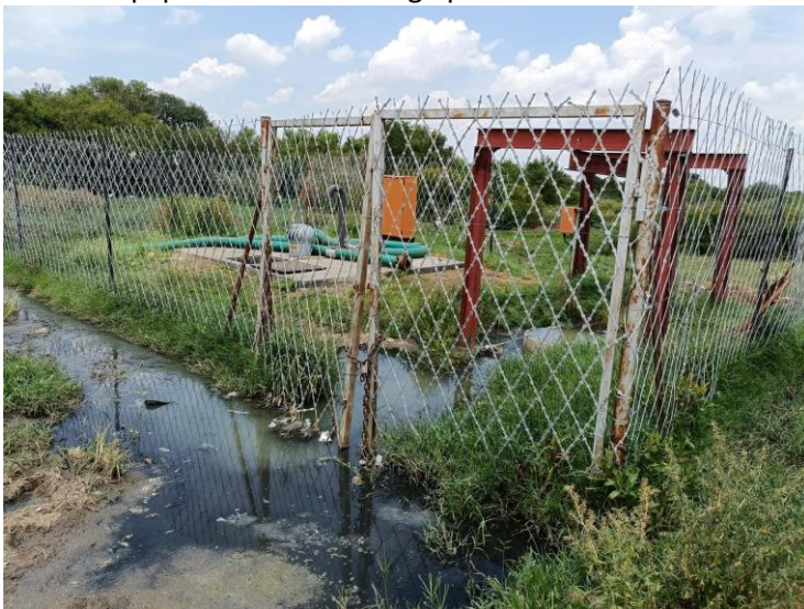
Raw sewage flowing into catchment areas and eventually the Vet River
