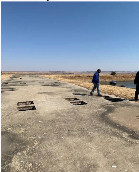
The waste water treatment plant in Ntha at Lindley was built and remains dysfunctional.
