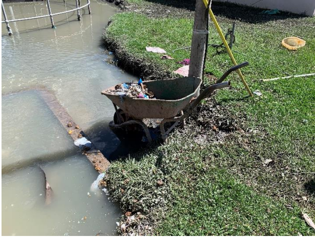
The waste water treatment plant that serves Mashaeng at Fouriesburg is dysfunctional with raw sewage flowing through streams into the Little Caledon and eventually the Caledon River.
