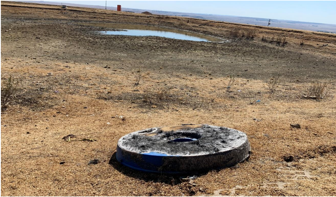
The waste water treatment plant in Ntha at Lindley was built and remains dysfunctional.
