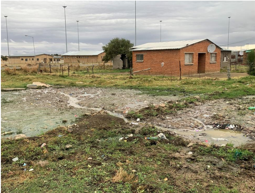
Raw sewage polluting streets in Makeleketla in Winburg
