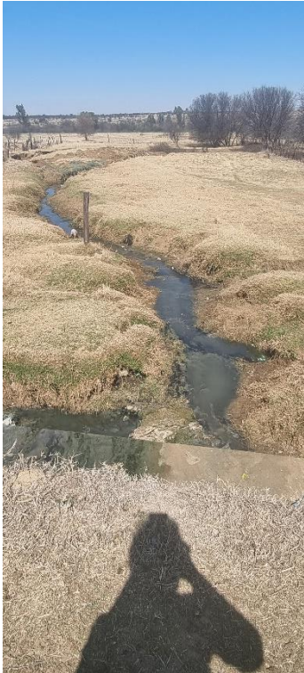
Sewage flows into streets, storm water systems and eventually the Vals River at Bothaville
